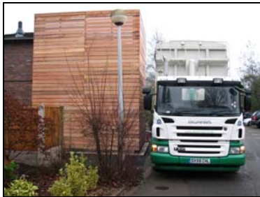
Delivering wood pellets to a HOVAL pellet boiler at a Telford Primary school.
