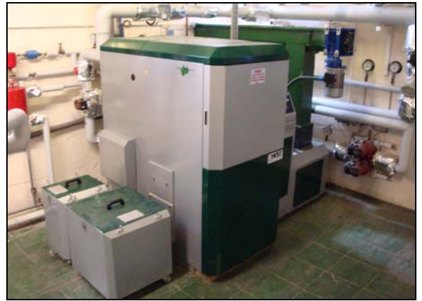
Several HERZ wood chip boilers installed by Rural Energy Ltd , at properties in Worcester, Crewe, Coventry and the Wyre Forest
